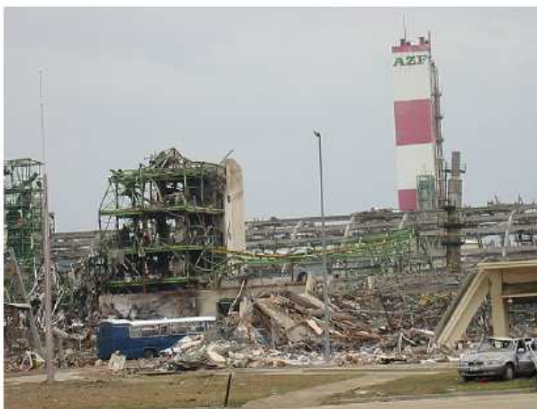
Fig 5. View of the AZF chemical plant after the explosion [12]
