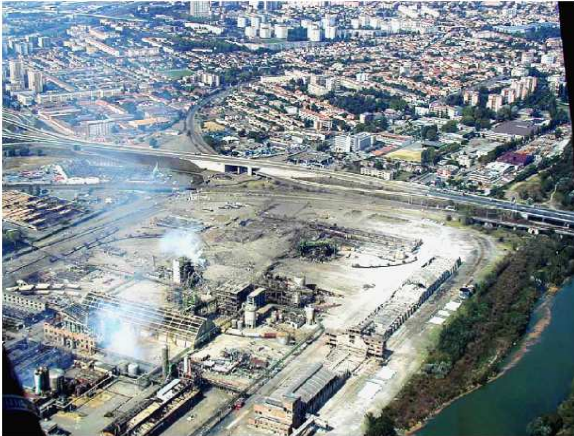
Fig 6. Effects of the AZF plant and nearby Toulouse city [13]
