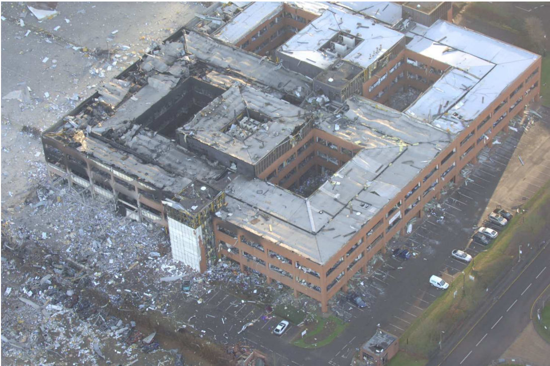
Fig 3. Damaged buncefield site. [8]
